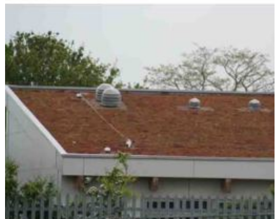
An example of a 'green' Sedum roof
