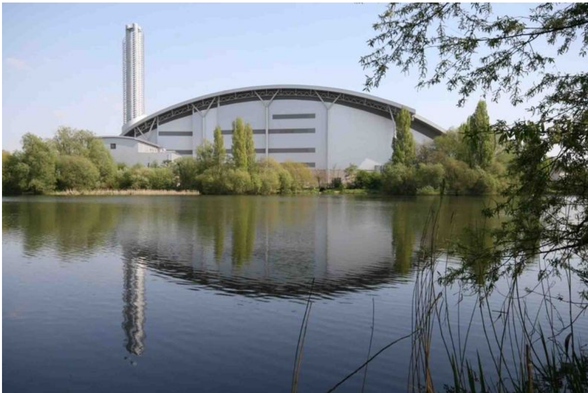
Energy from Waste Facility Lakeside (Grundon)
