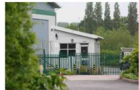
A simple gatehouse, but let down by the utilitarian security gates
