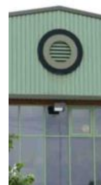
Ventilation should be incorporated into facade design
