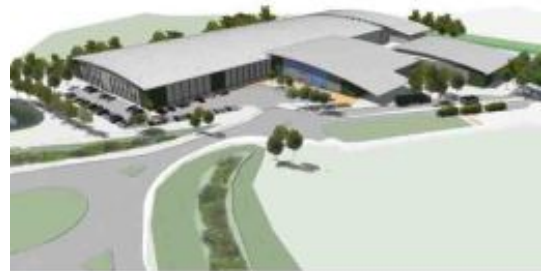
A good example of built form
