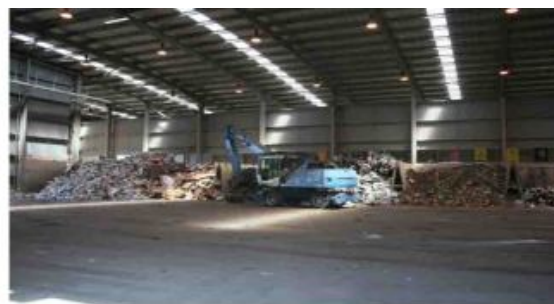
The 'operational' side of a Household Recycling Facility
