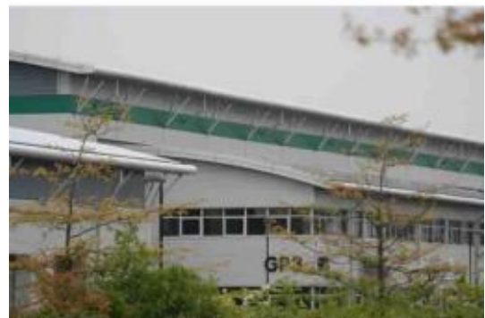
Offices on the side of the building can add interest to the built form
