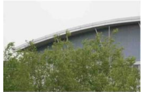
Curved roofs can provide interest
