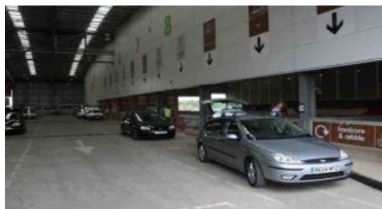
Internal view of a Household Recycling Facility
