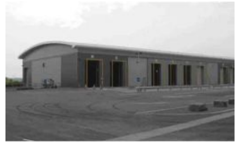
Built form of Alconbury Waste Transfer Station
